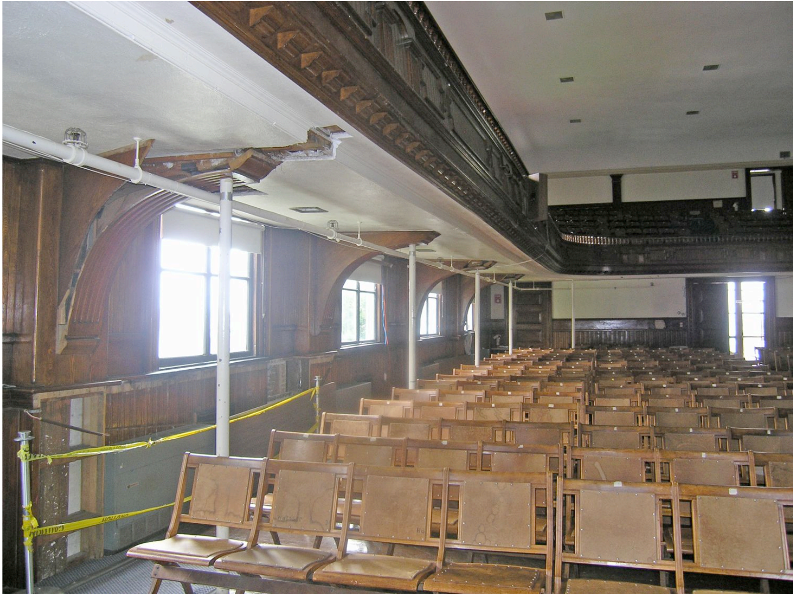
Auditorium with Shoring below Each Balcony Level
