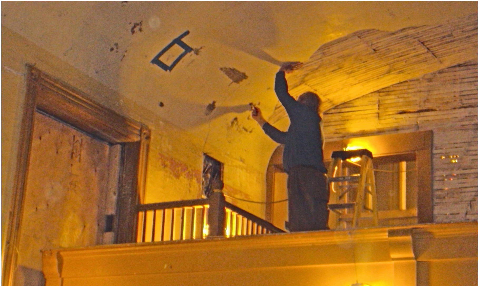
Andrew Ladygo, Architectural Conservator, Exposing the Original Ceiling Stenciling
