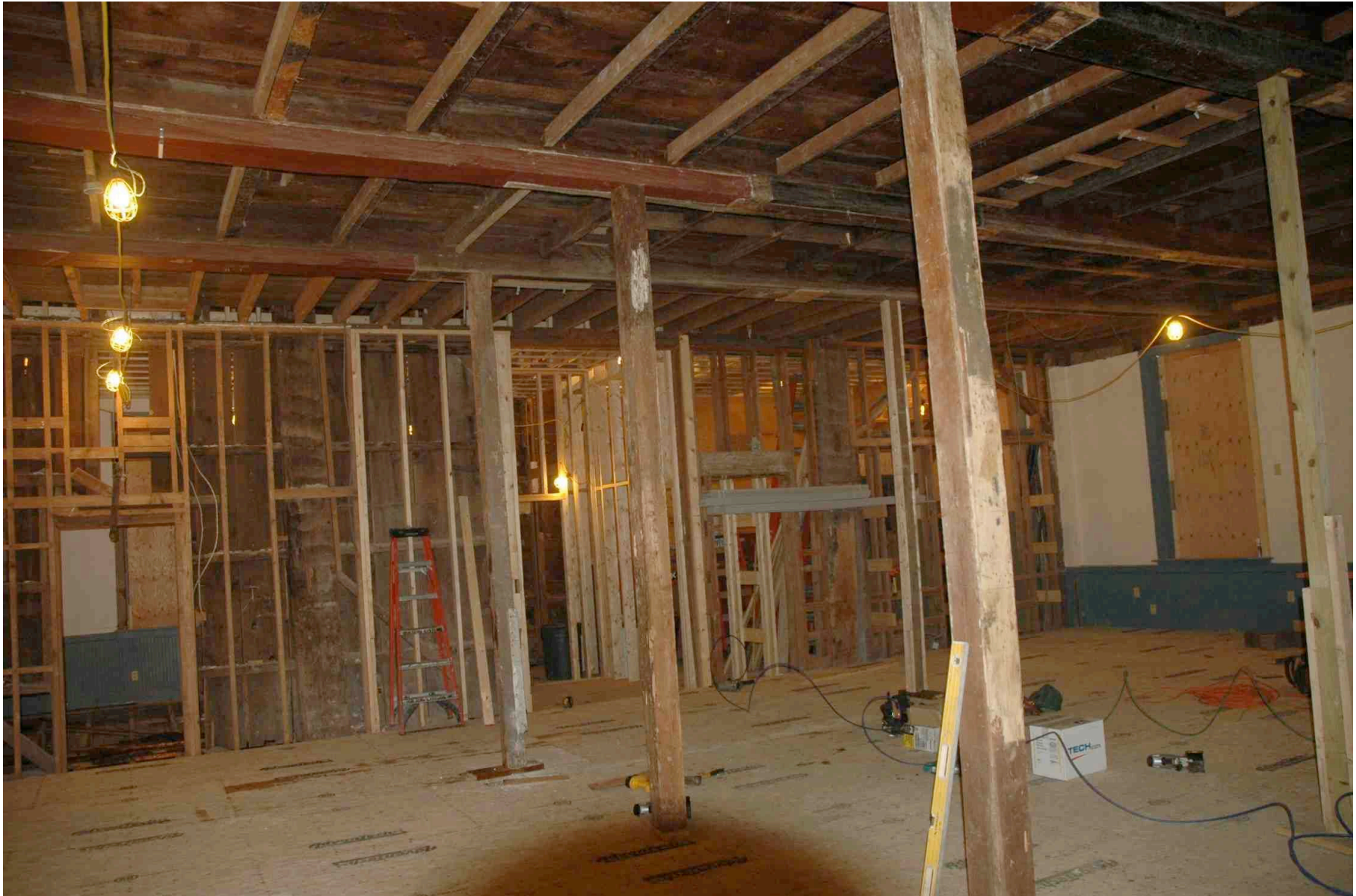
Structural Reinforcement of Second Floor Framing
