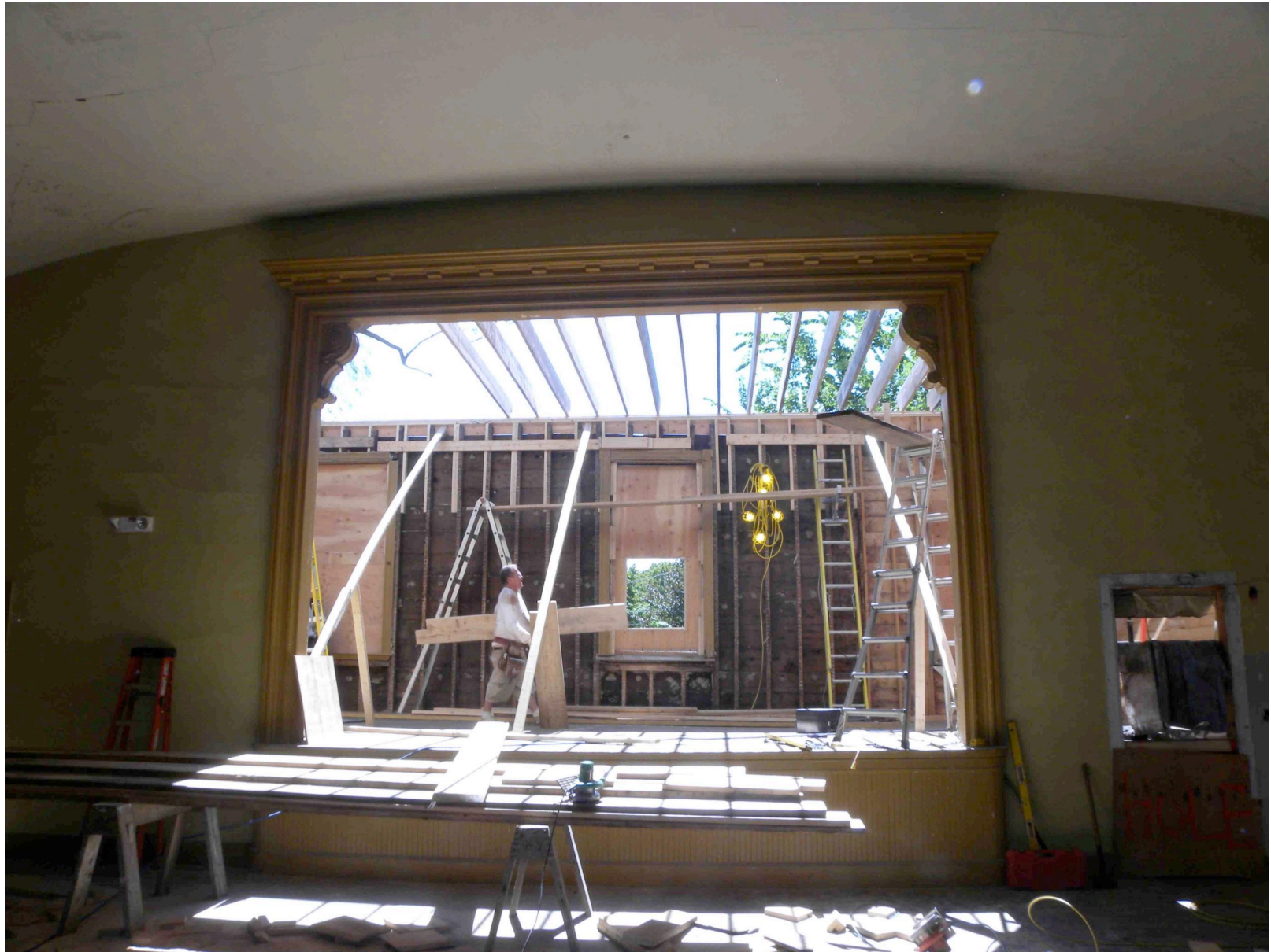
Reframing of the Stage Roof
