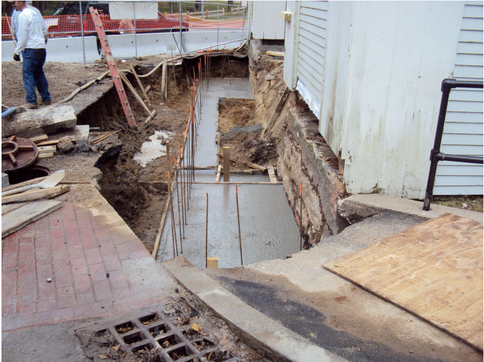
New Footing for Accessible Sloped Walk in Front of Town Hall
