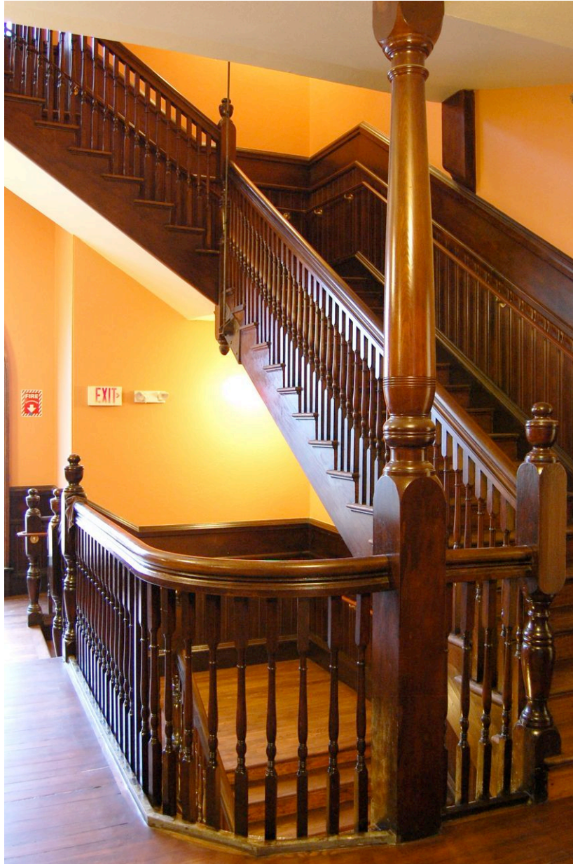
View of Stair from Auditorium to Balcony
