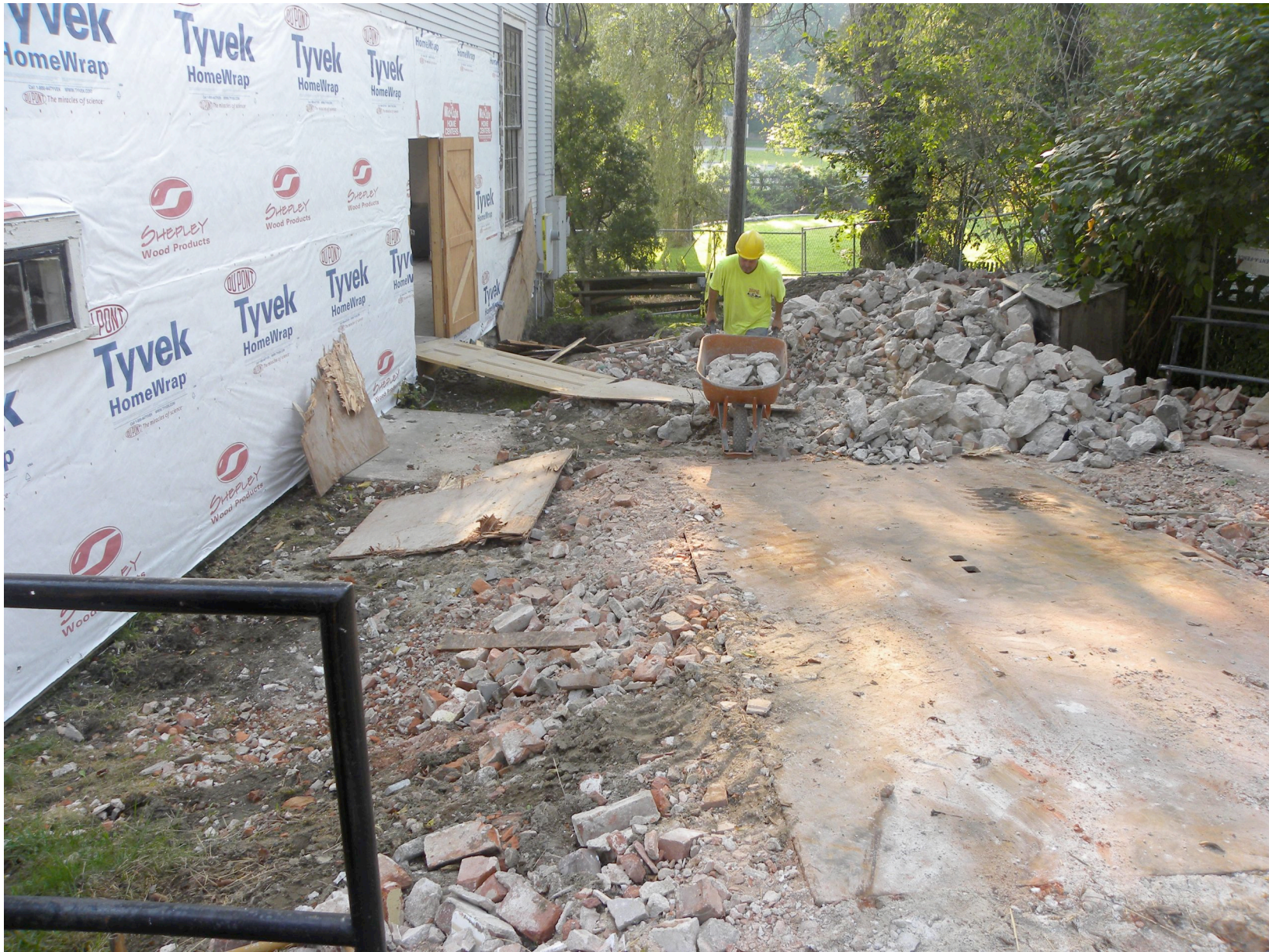
Removal of Vault Foundation Walls
