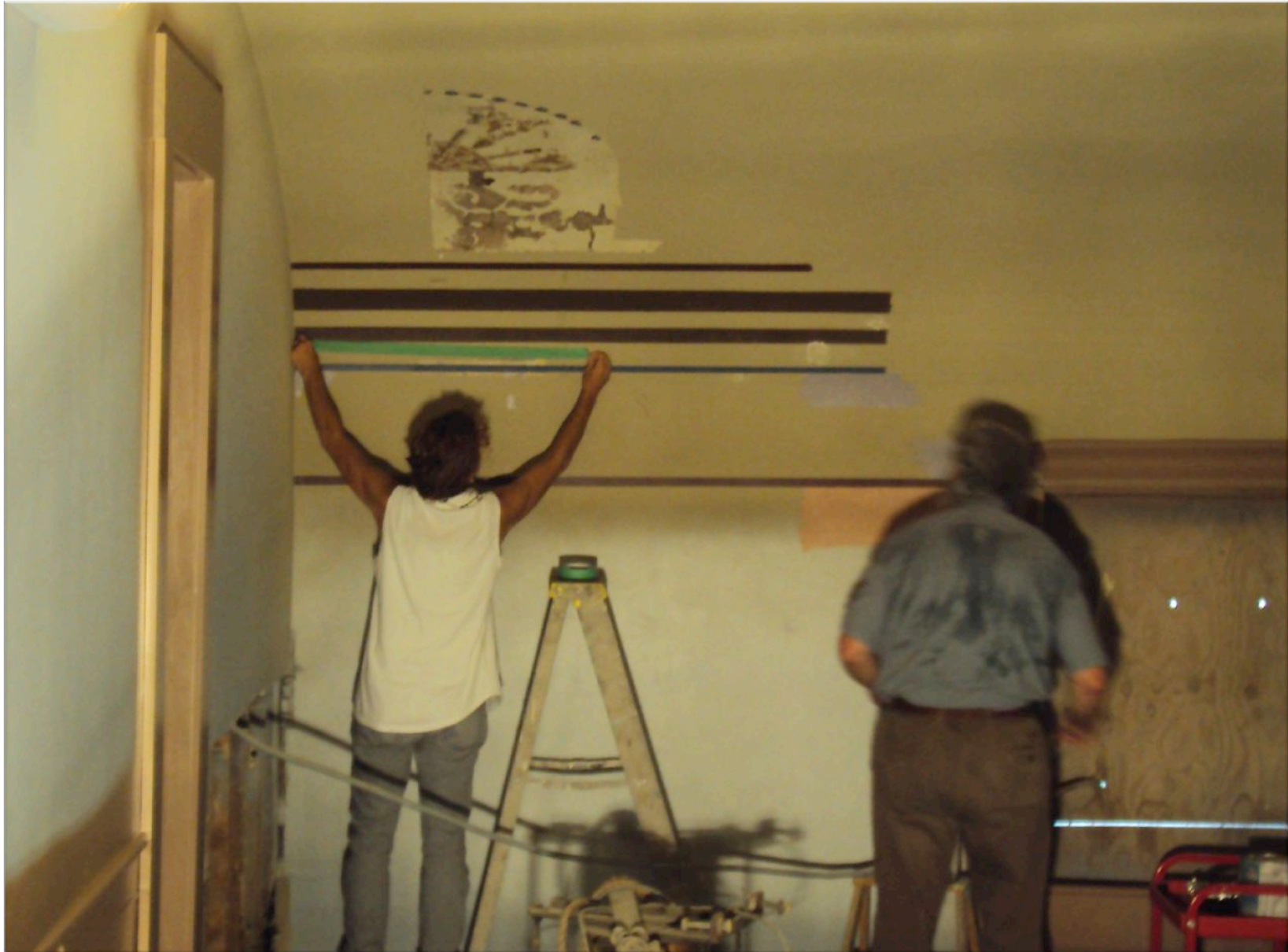
Sharon Perlmutter and Andrew Ladygo Starting to Replicate Original Stenciling
