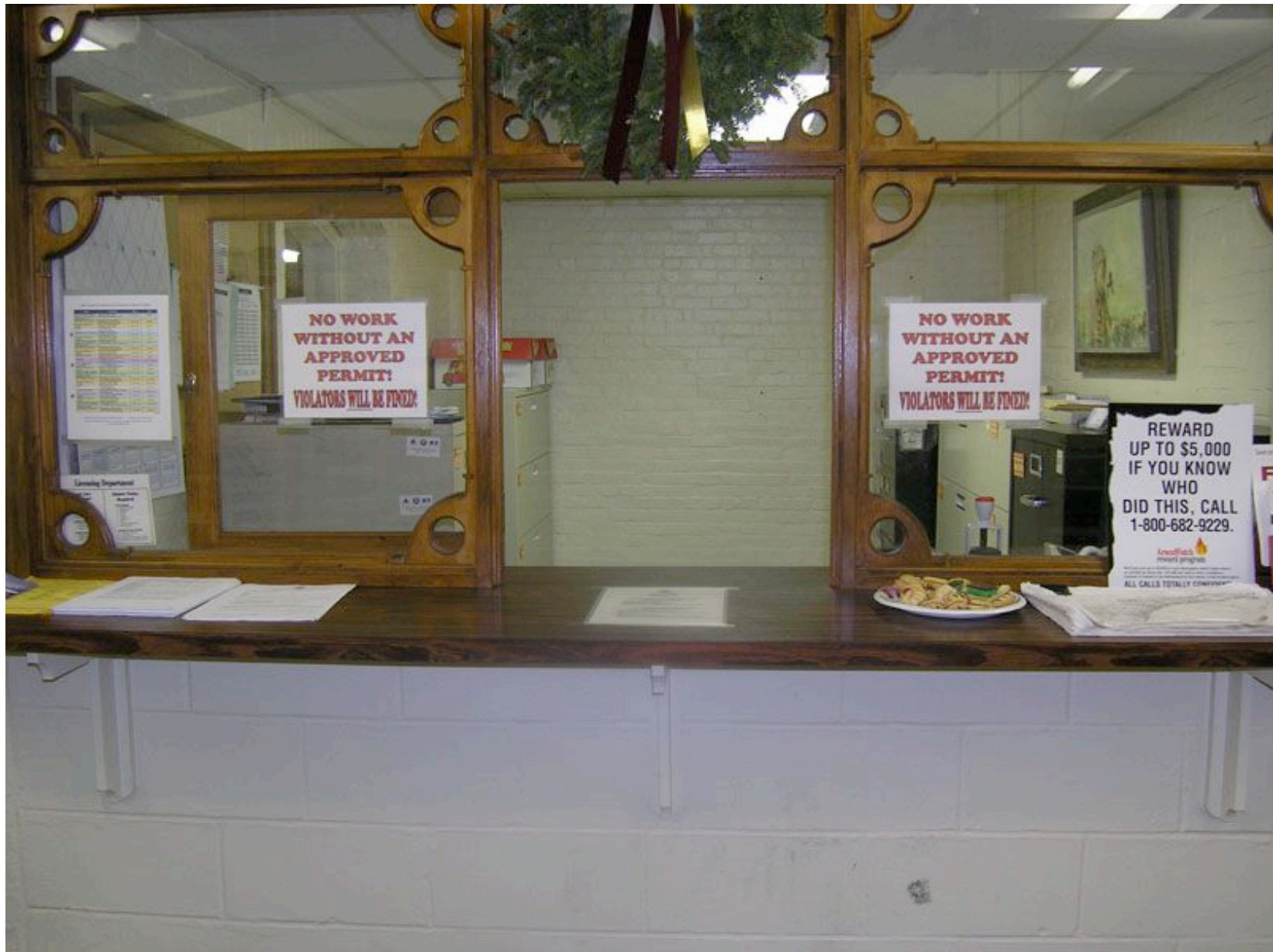
Pre-Restoration Photograph of Municipal Counter on Ground Floor
