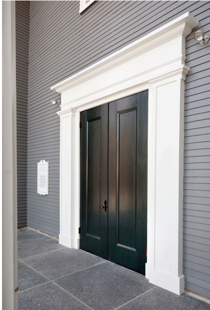
Restored and Fully Accessible Entry Doors
