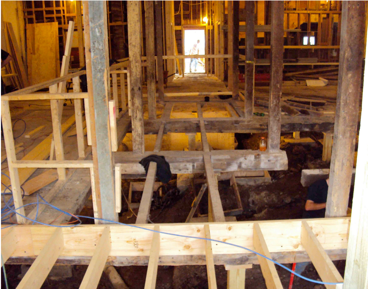
First Floor Structural Repairs
