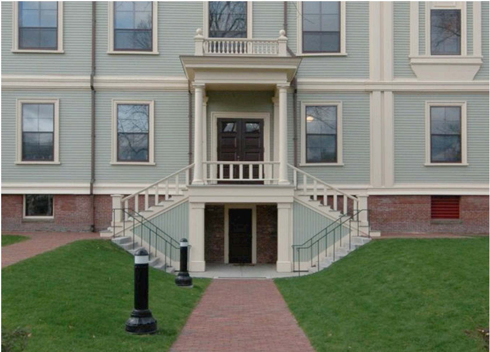
Completed Fully Accessible Provincetown Town Hall Ryder Street Entry
