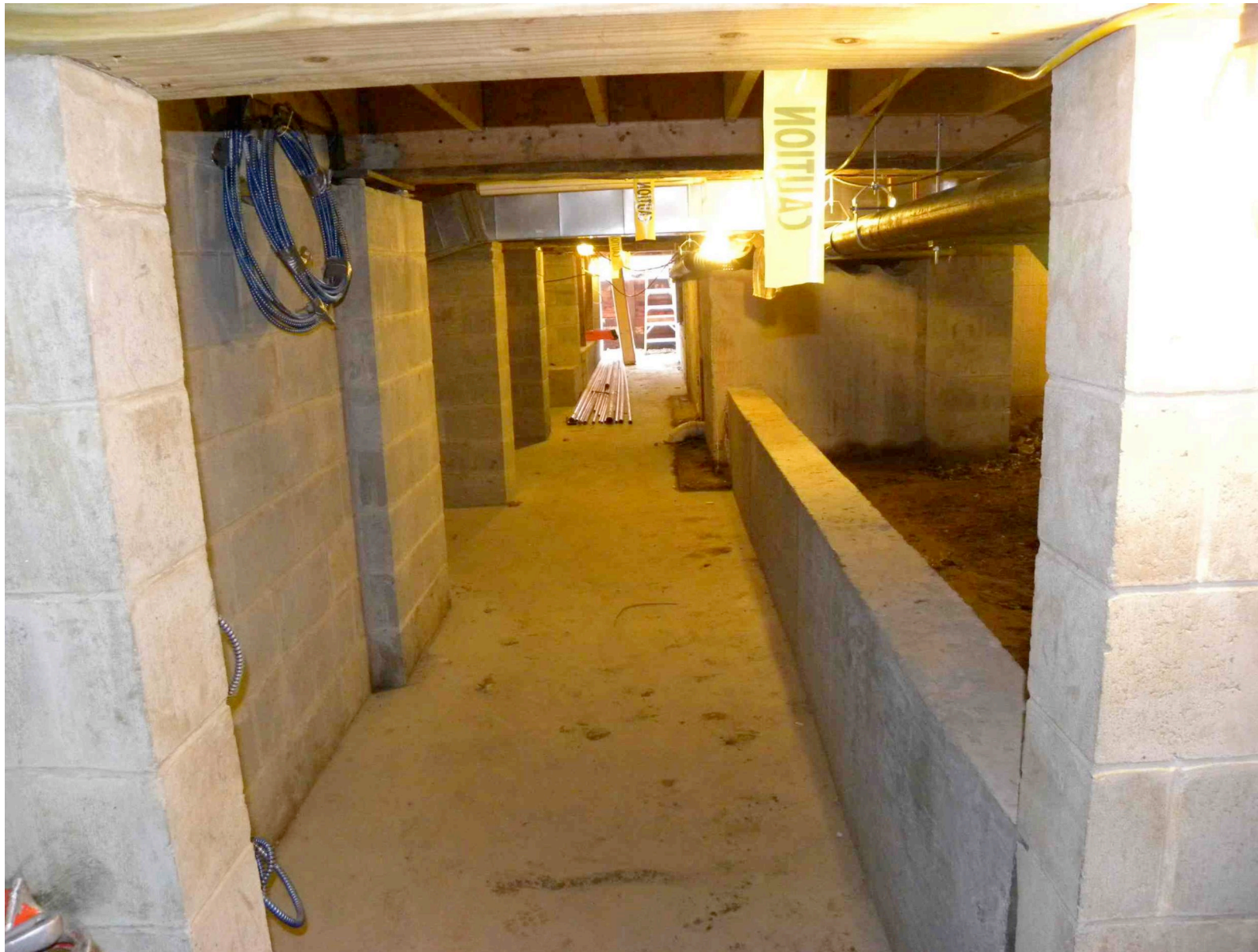
New Basement Access to Mechanical Area
