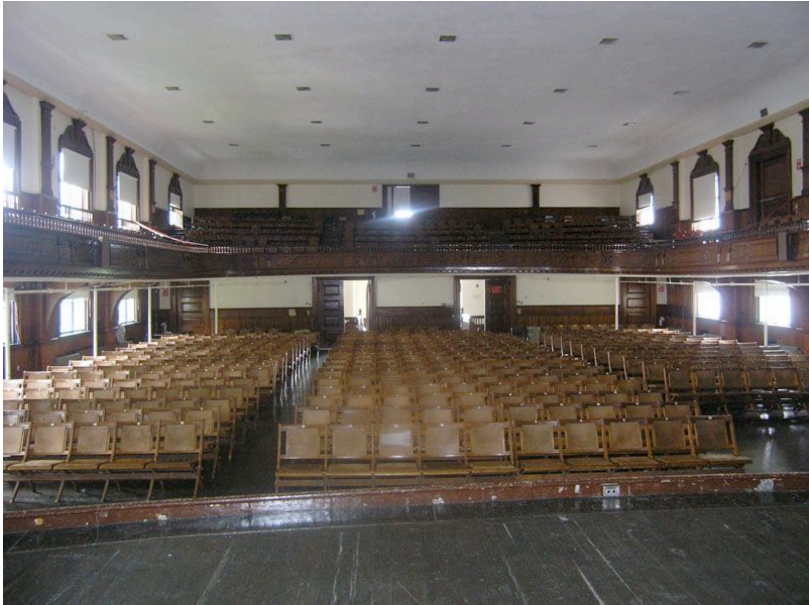
Pre-Restoration View of Auditorium Looking Toward Balcony from Stage
