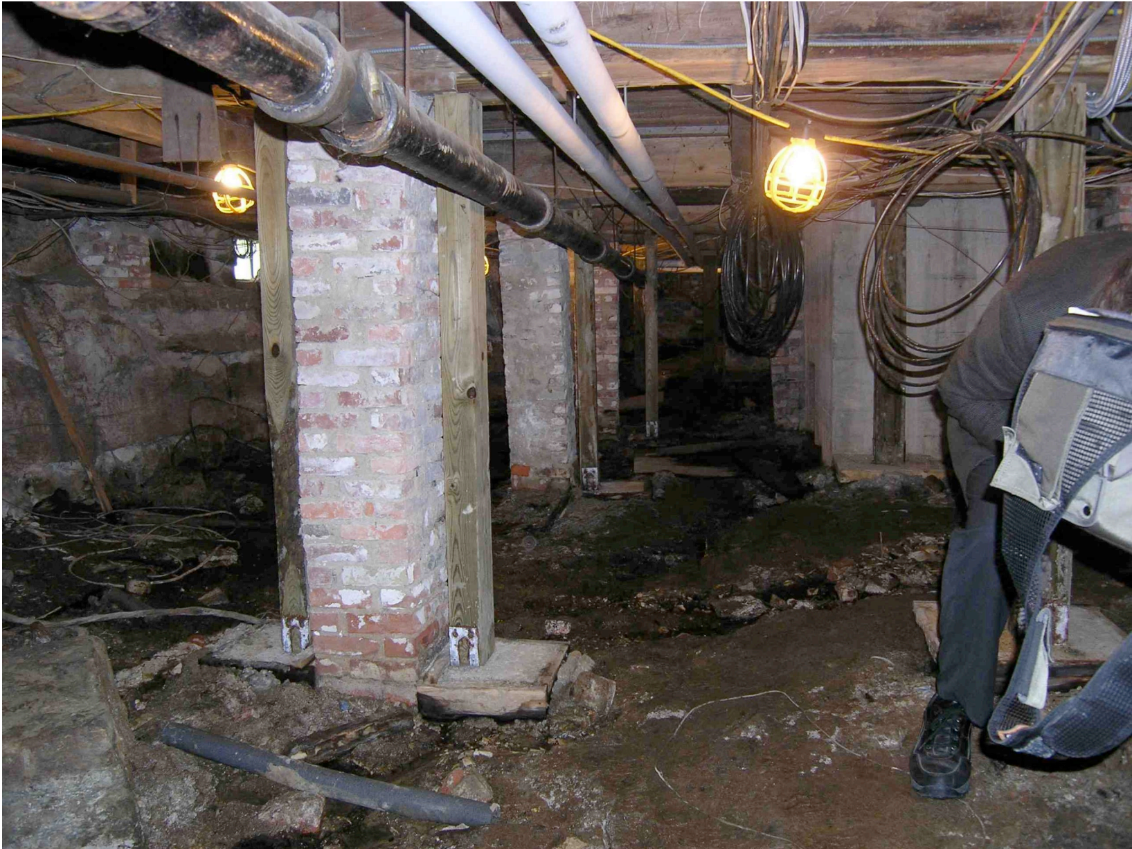
2008 View of Basement
