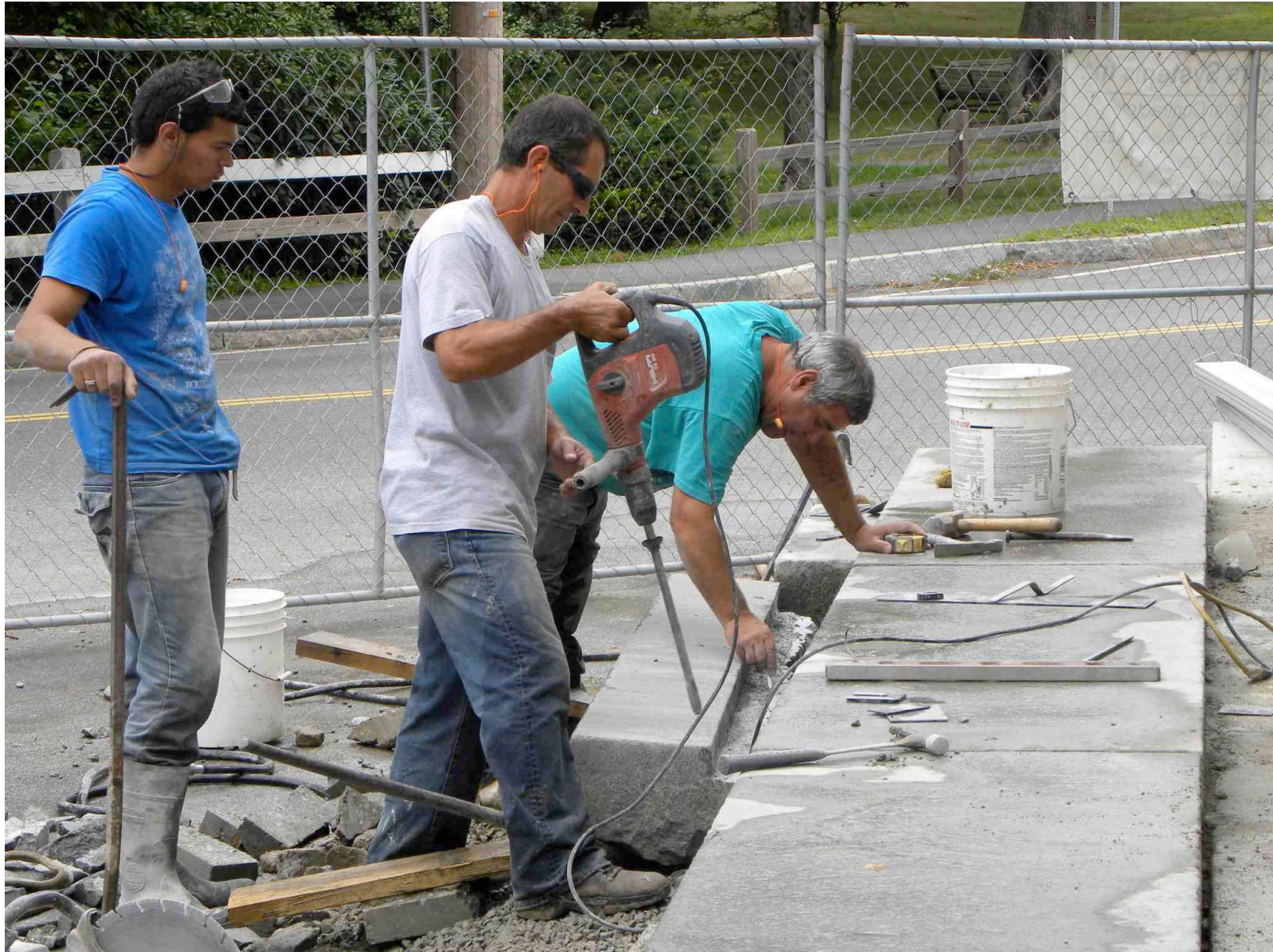
Reinstallation of Original Granite Steps
