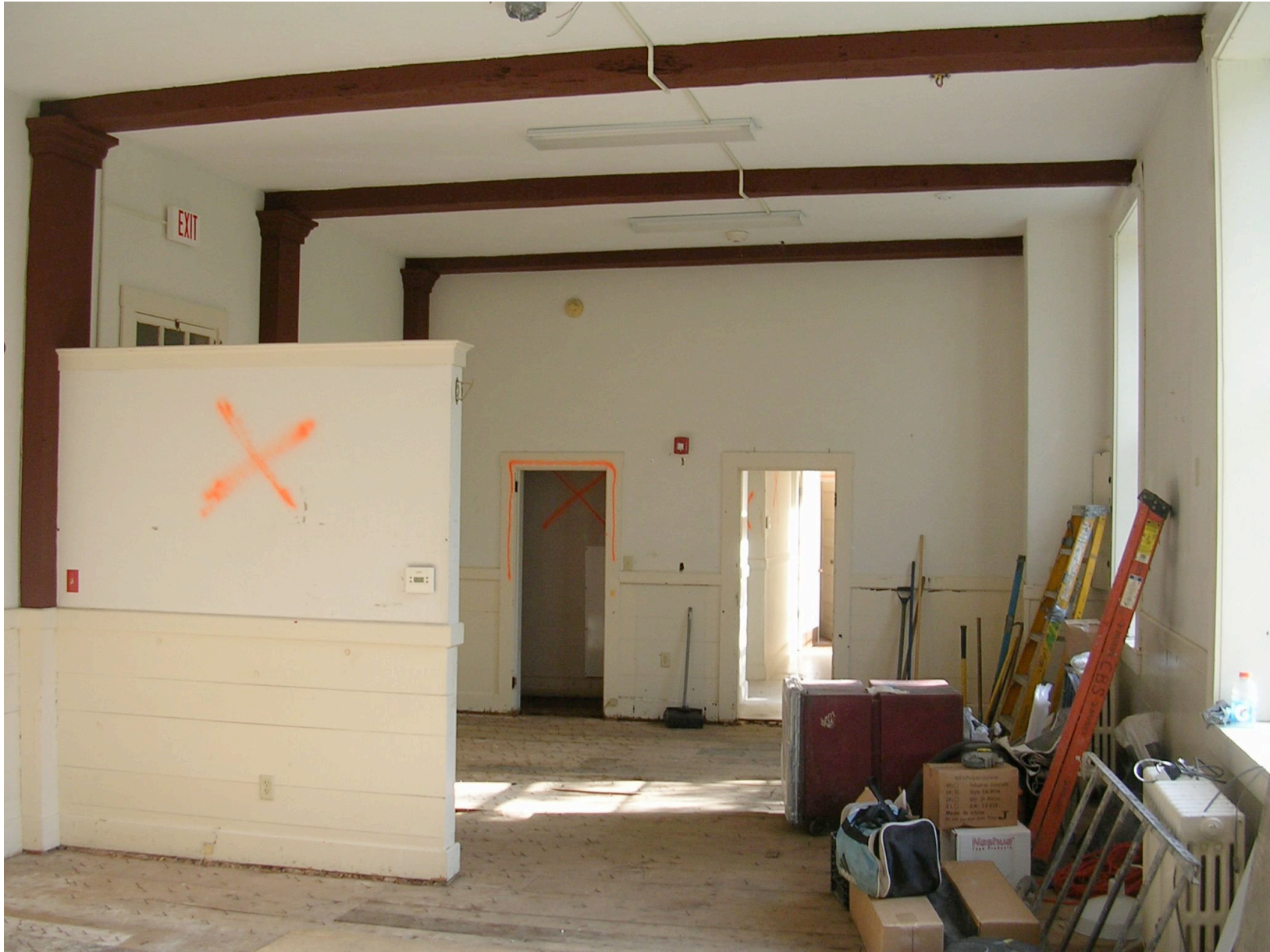
First Floor Interior at Start of Construction
