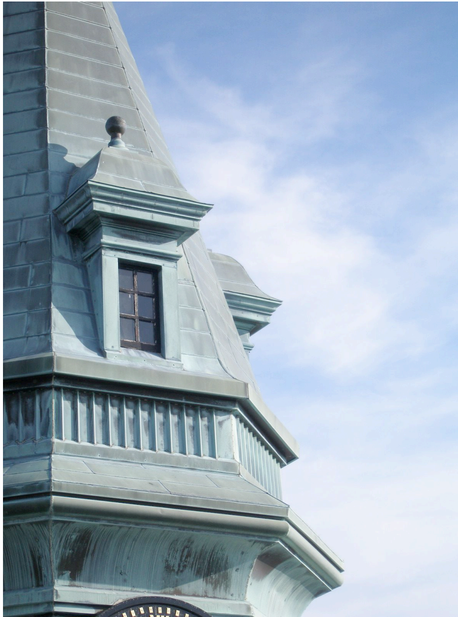
Closeup View of Lantern Level of Copper-Clad Clock Tower
