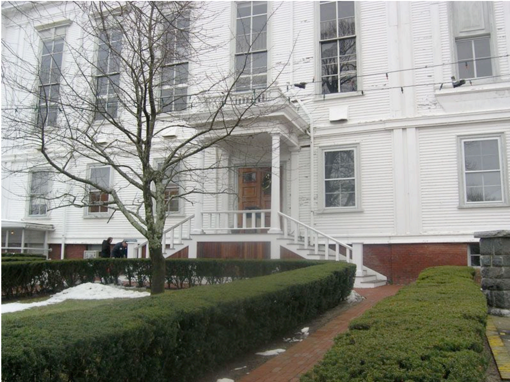
Pre-Restoration Photograph of Provincetown Town Hall Ryder Street Entry
