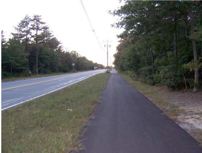
Figure 2.4-24: Forest Road Path, Looking North
