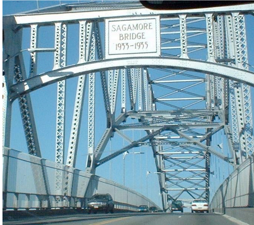
Figure 2.8-3 - Roadway over Sagamore Bridge
