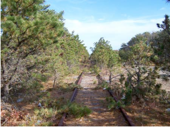
Figure 2.5-15: Rail Tracks East of Station Avenue in Yarmouth
