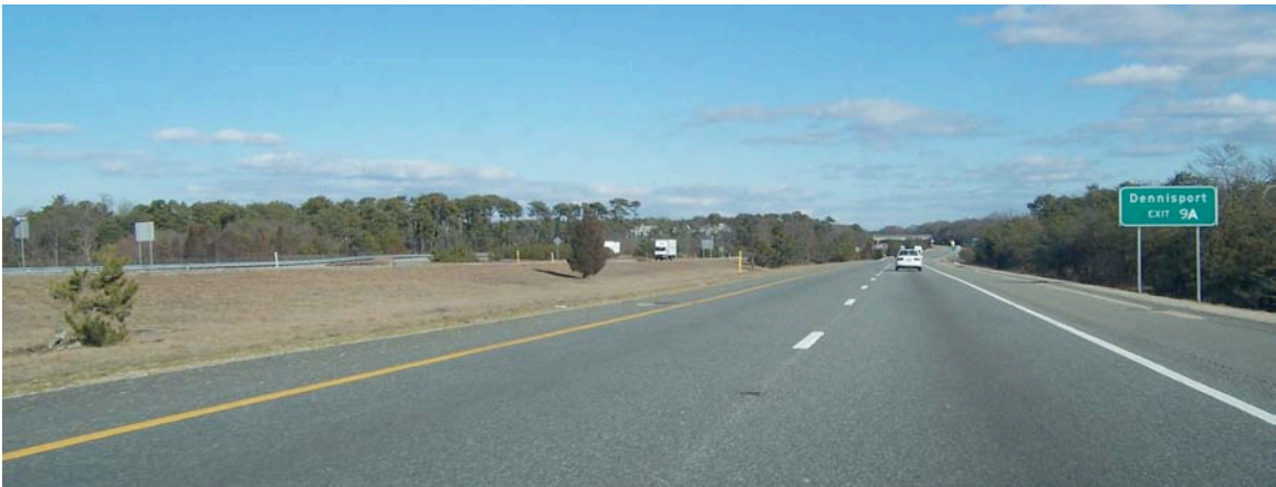
Figure 2.2-26 - Route 6 between exits 8 and 9 (Mid-Cape)
