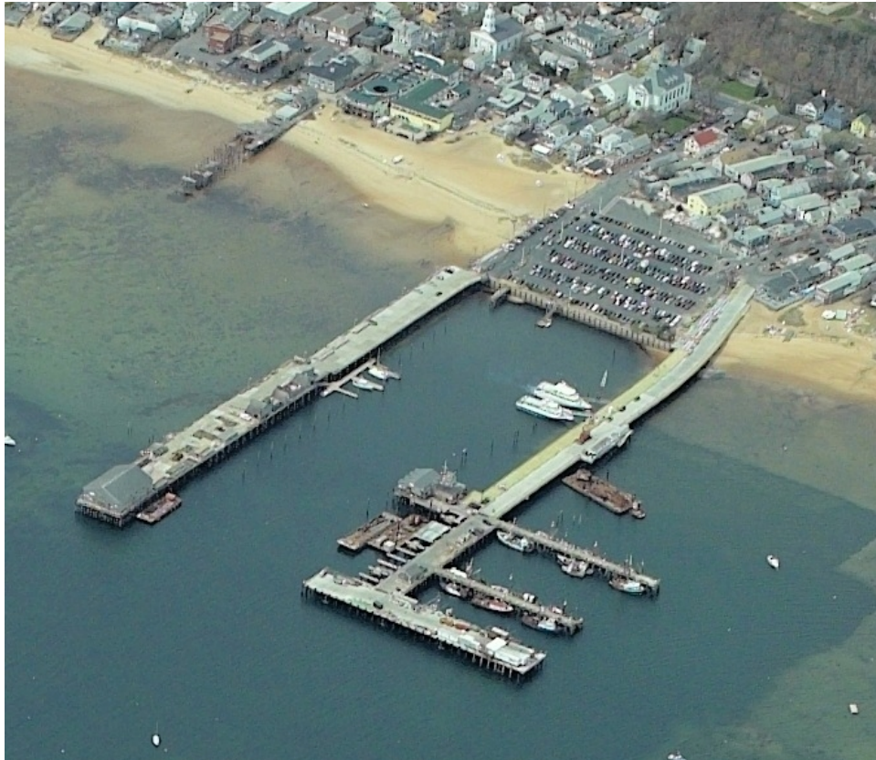
Figure 2.3-7: Aerial View of the MacMillan Pier in Provincetown
