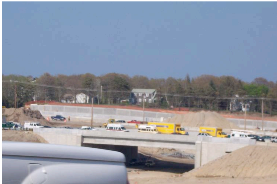
Figure 2.8-21 - The Sagamore Interchange overpass, during construction
