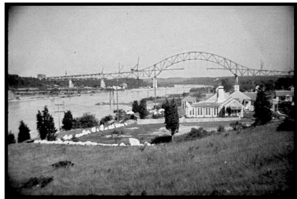
Figure 2.6-17: Construction of the Bourne Bridge 19
