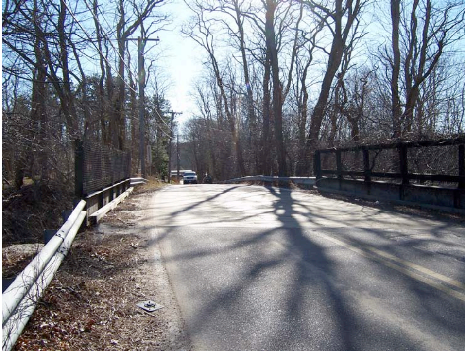
Figure 2.2-22 - The Northern Crossing of Palmer Avenue over the Bay Colony Railroad Tracks in Falmouth
