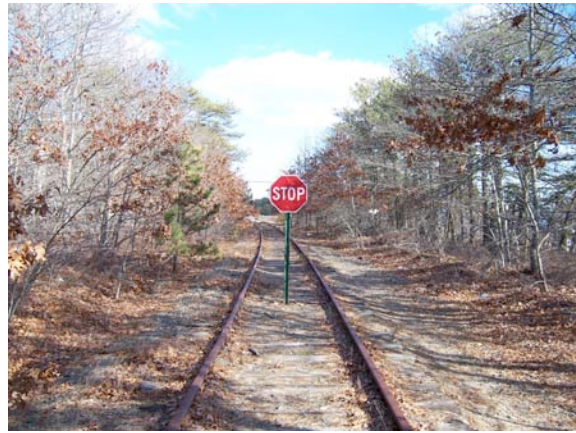
Figure 2.5-14: Rail Tracks in Yarmouth West of Station Avenue.
