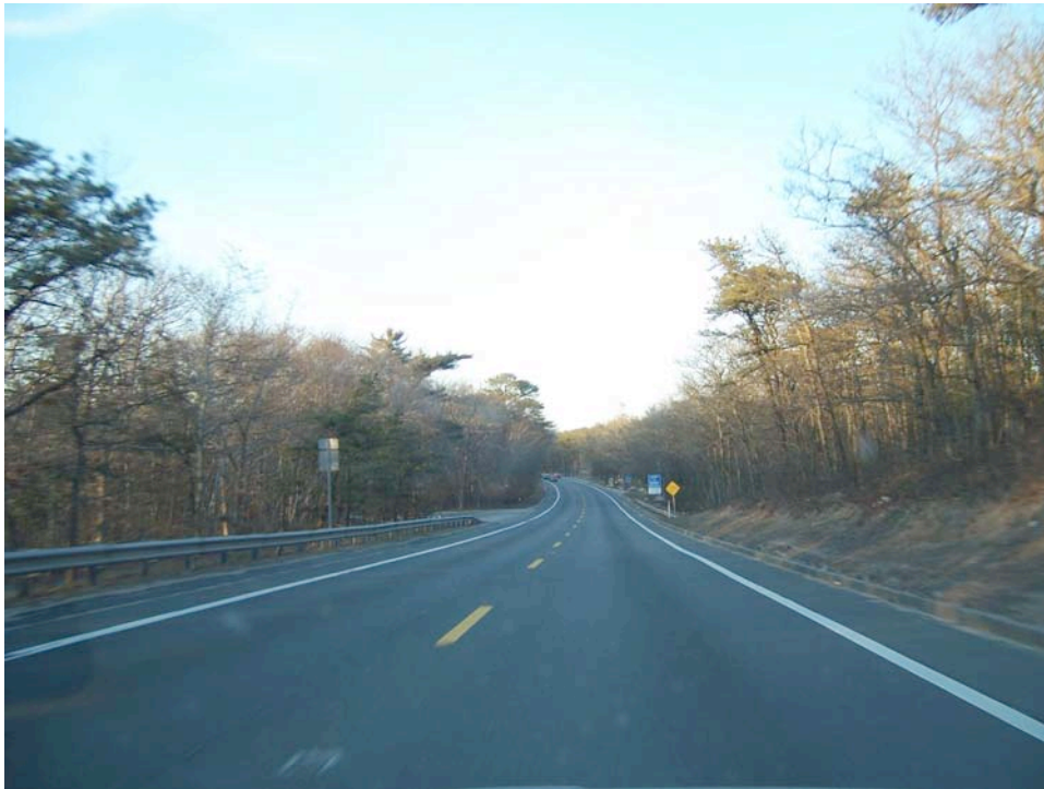
Figure 2.8-15 - Sandwich Road facing East
