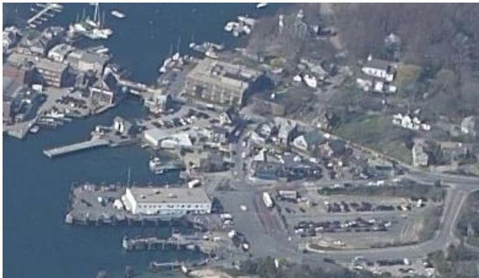
Figure 2.3-8: Aerial View of the Steamship Authority Piers in Woods Hole
