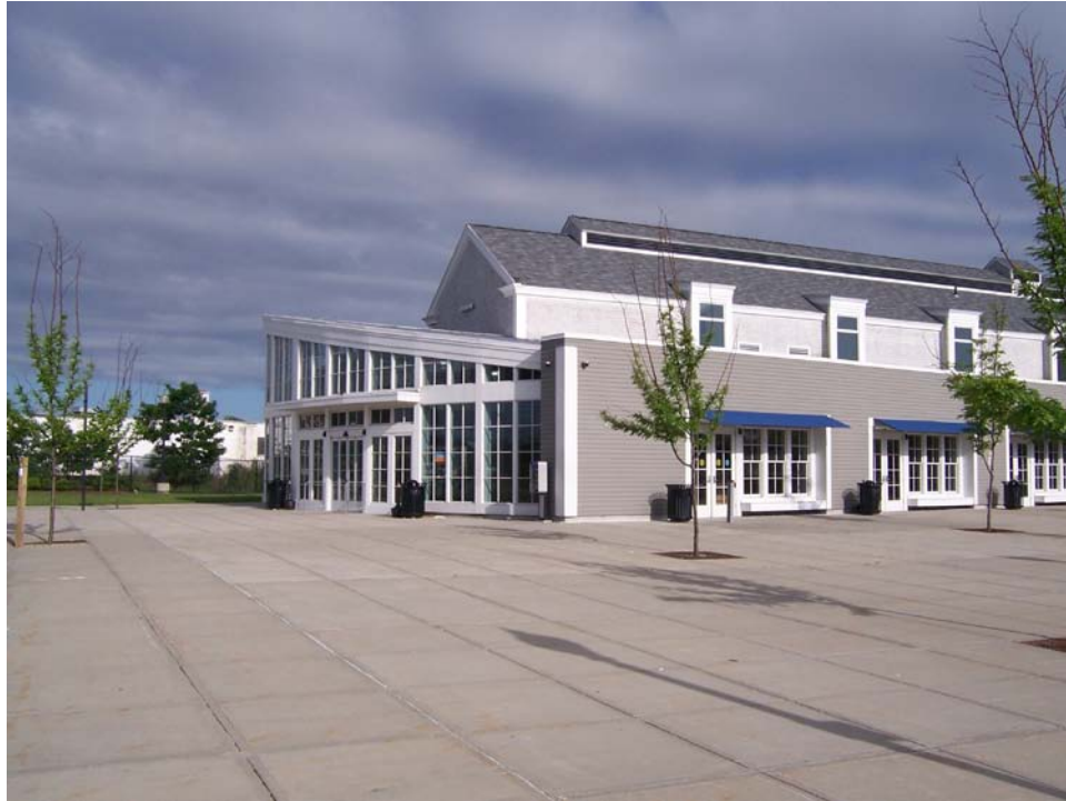
Figure 2.3-4: Hyannis Transportation Center, West Side
