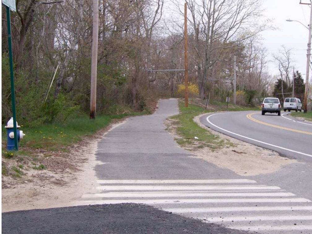
Figure 2.4-18: Looking North on Route 130 Bicycle Path at Lovell's Lane, Mashpee
