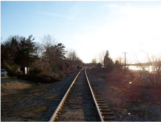
Figure 2.5-7: Rail Tracks West of the Sagamore Bridge
