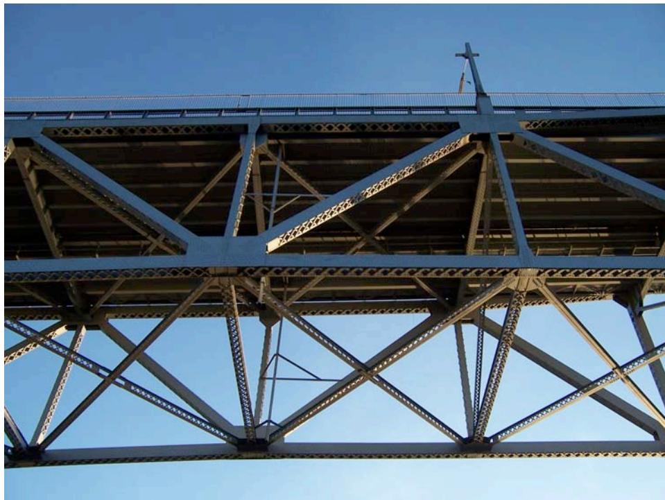
Figure 2.8-4 - Sagamore Bridge Structure
