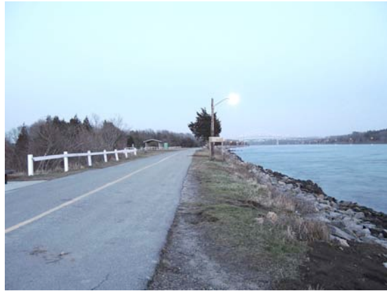
Figure 2.4-8: Mainland-Side of the Canal Bicycle Path, East of Railroad Bridge
