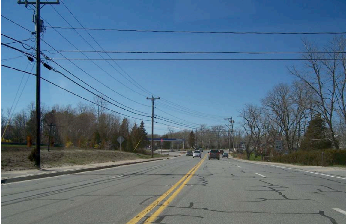
Figure 2.2-28 - Route 6 North of Governor Prence Road, Eastham (Outer Cape)
