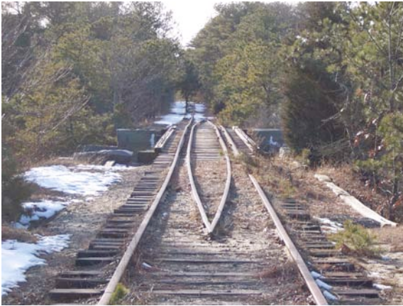
Figure 2.5-17: Bass River Rail Bridge, Facing West
