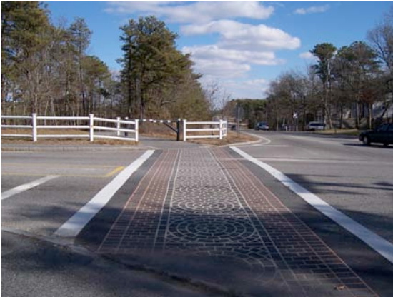
Figure 2.4-31: West Yarmouth Road crossing of the Old Townhouse Road Trail
