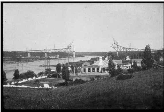
Figure 2.6-16: Construction of the Bourne Bridge 18
