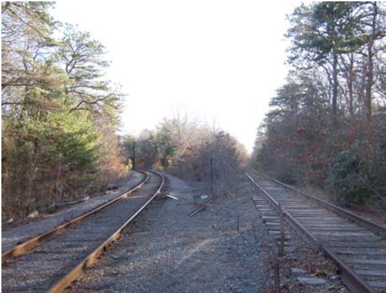
Figure 2.5-22: Rail Tracks at the Otis Junction.
