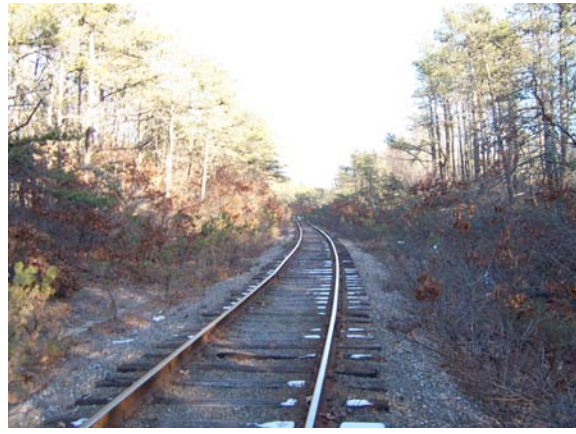
Figure 2.5-27: Otis Branch Rail Tracks, East of Route 28A
