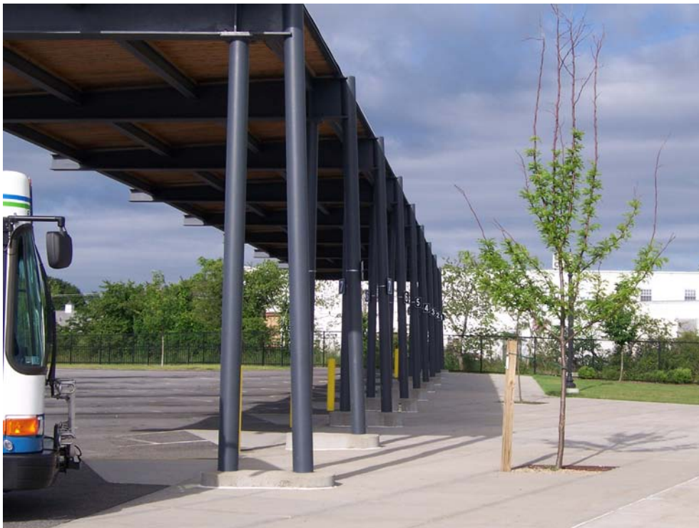
Figure 2.3-5: Bus Terminal at the Hyannis Transportation Center
