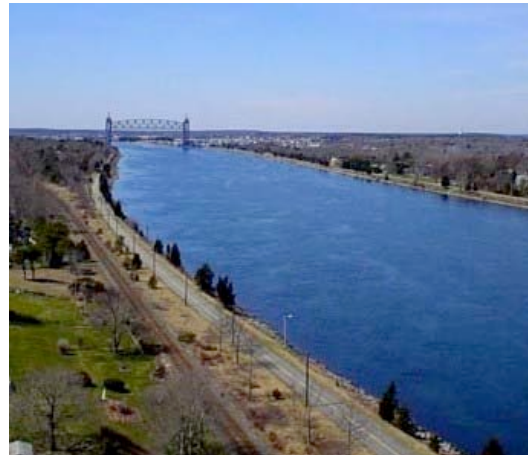
Figure 2.6-19: Cape Cod Canal and Railroad Bridge in the distance, facing west
