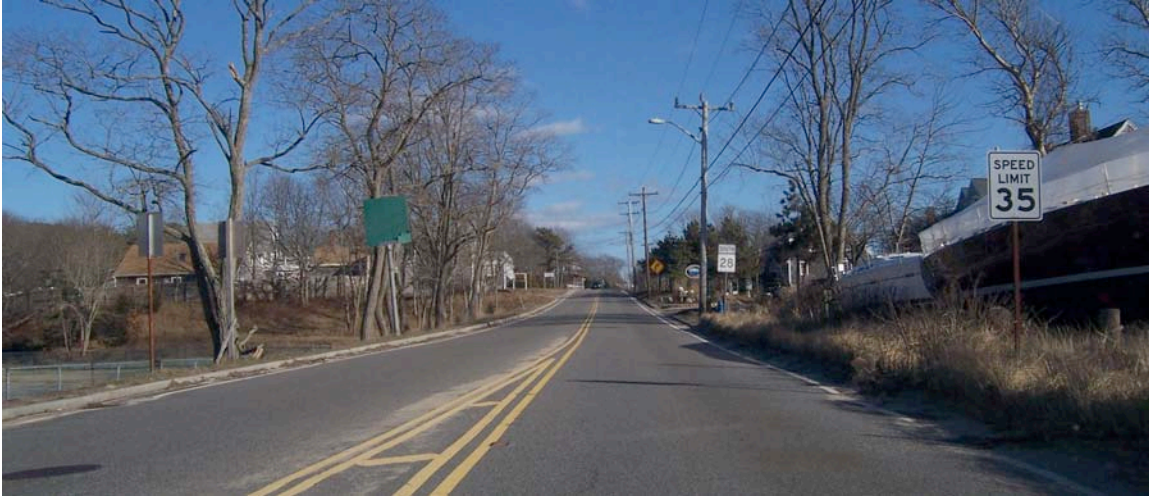
Figure 2.2-33 - Route 28 east of Routes 124 and 39 (Lower Cape)
