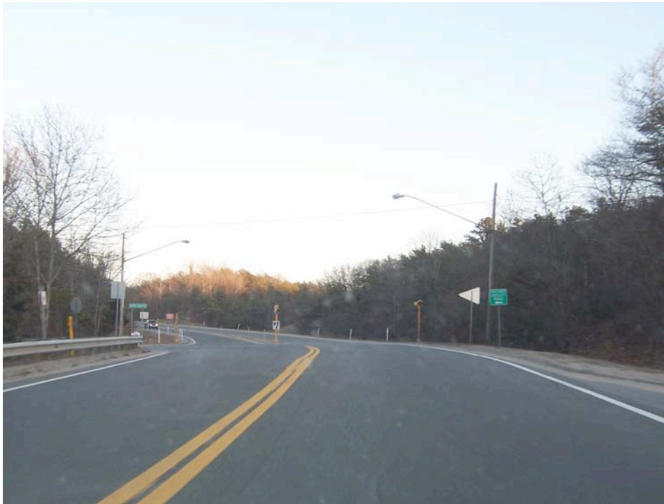
Figure 2.8-22 - The Mid-Cape Connector (Interchange 1) north of the Outlet Store entrance
