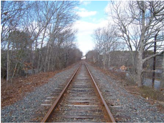
Figure 2.5-19: Rail Tracks West of Willow Street, Facing North
