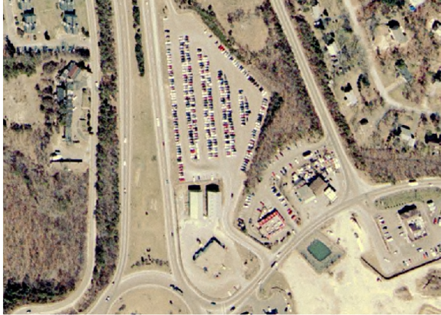
Figure 2.3-9: Aerial View of the Original Sagamore Park-and-Ride Lot, 2002
