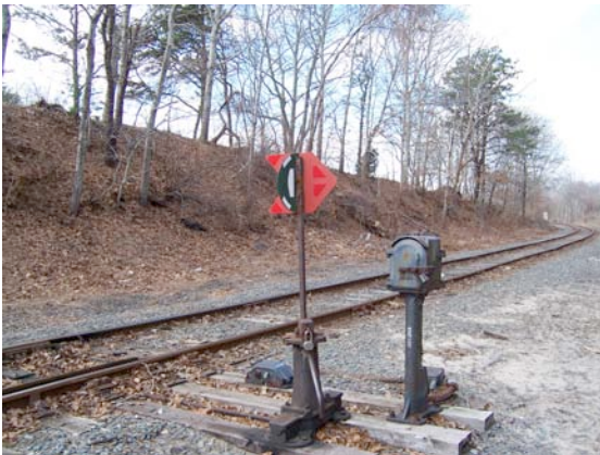
Figure 2.5-9: Rail Tracks and Switch West of Willow Street in Yarmouth
