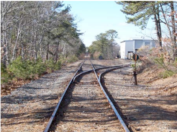
Figure 2.5-13: Rail Tracks in Yarmouth, Facing West.
