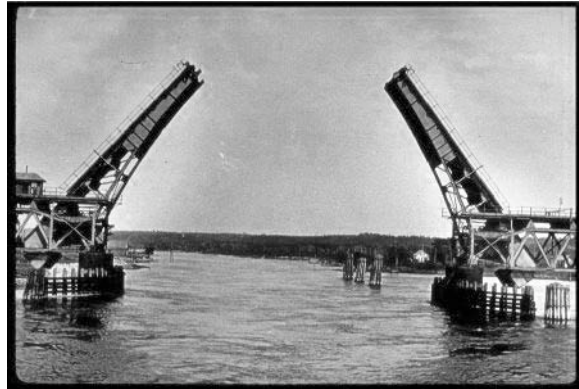
Figure 2.6-13: The original Bourne Bridge completed in 1911 15
