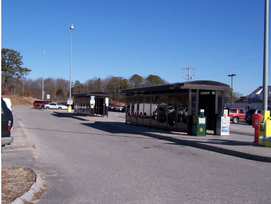
Figure 2.3-10: Bus Shelters at Barnstable Park-and-Ride Lot
