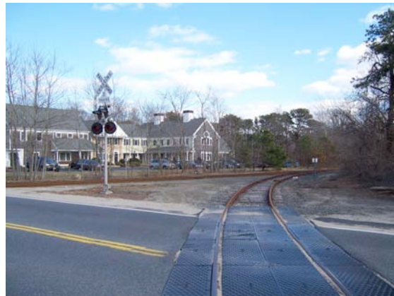
Figure 2.5-10: Rail Crossing at Willow Street in Yarmouth, Facing East
