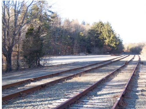
Figure 2.5-23: Rail Tracks North of Old County Road in Falmouth
