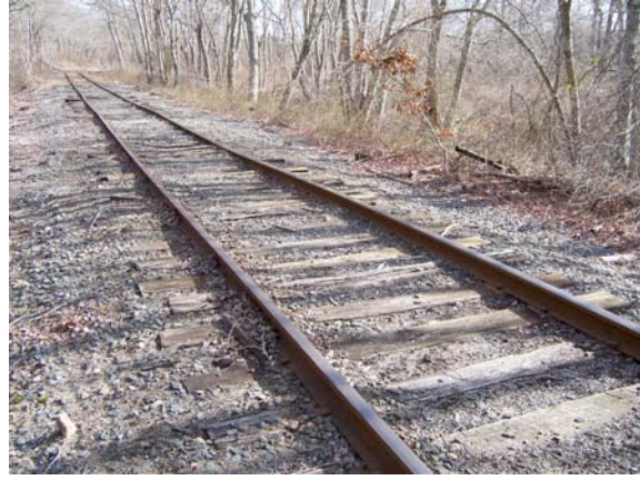
Figure 2.5-12: Rail Tracks East of Willow Street in Yarmouth
