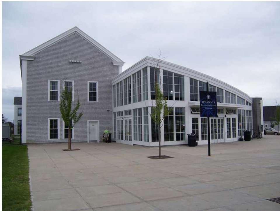
Figure 2.3-3: Hyannis Transportation Center, North Side
