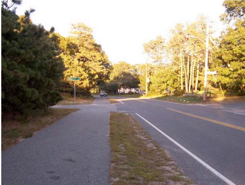
Figure 2.4-12: Setucket Road Path East of North Dennis Road, Looking East
