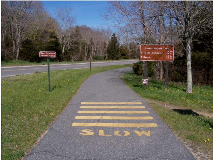
Figure 2.4-15: Nauset Trail from the Salt Pond Visitor’s Center Looking East
